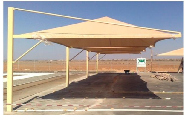
Fig. 1. Typical vehicle shade: steel cantilever frame with stretched fabric canopy [1].
