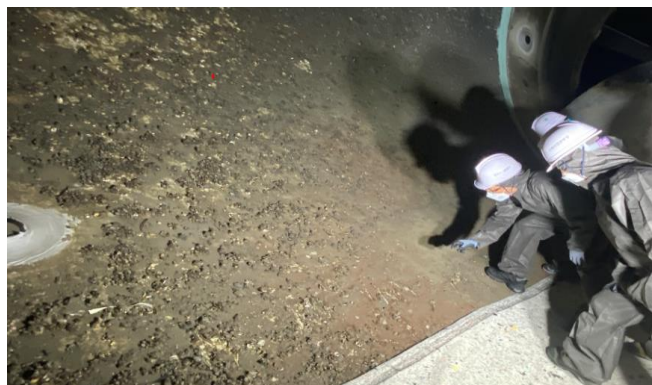
Fig. 6. Attachment of barnacles to draft tube liner.
