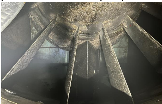
Fig. 4. Attachment of barnacles to wicket gates.
