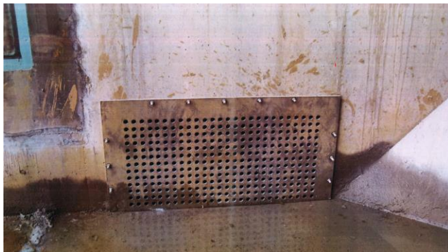
Fig. 2. Drainage screen. There is a drainage screen on the wall below the seawater inlet. During a major inspection, the water in the aqueduct is drained through this drainage screen, but this is difficult due to the adhered mussels.
