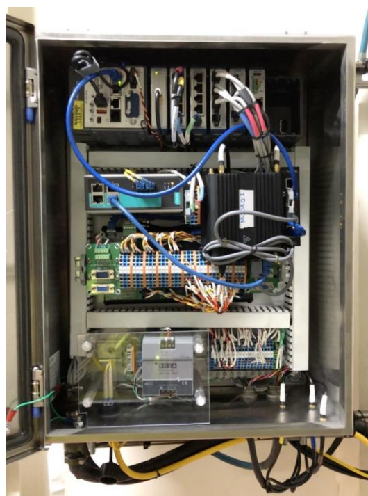
Fig. 6 Enclosure layout of a MODAQ field enclosure (Photo by Robert Raye, NREL)
