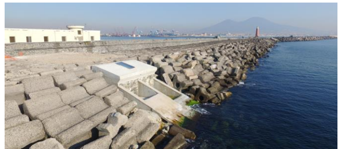
Fig. 2. Overtopping Breakwater for wave Energy Conversion prototype
