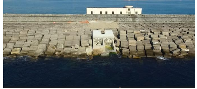
Fig. 1. Photo of the OBREC device integrated in the existing breakwater of the San Vincenzo pier in the port of Naples (Italy).
