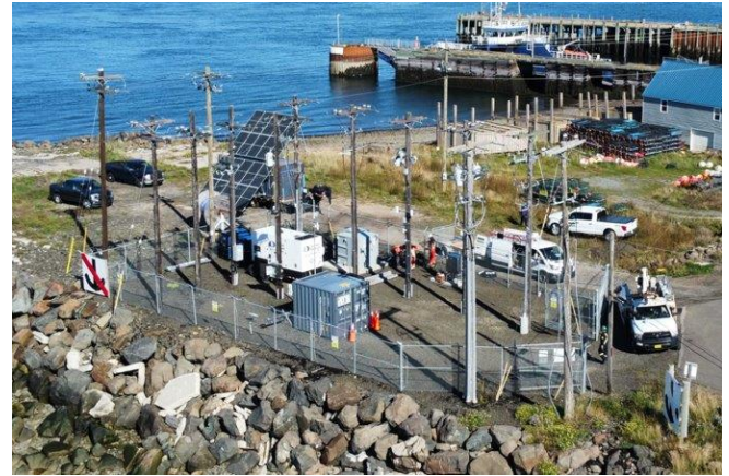
Fig. 5: Land-based substation with pole infrastructure, transformer and control container housing switch gear, communication basis and SCADA system.
