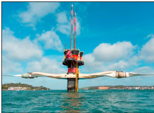
Fig. 1. SeaGen Tidal Turbine installed in Strangford Lough, Northern Ireland. The first commercial scale grid connected tidal turbine in the world.
