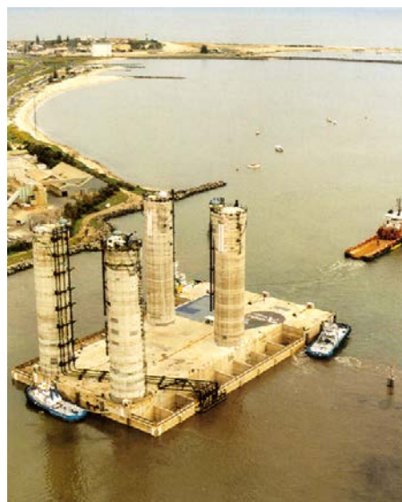
Fig. 1. Wandoo Concrete Gravity Structure during tow-out of a casting basin in Western Australia [1].
