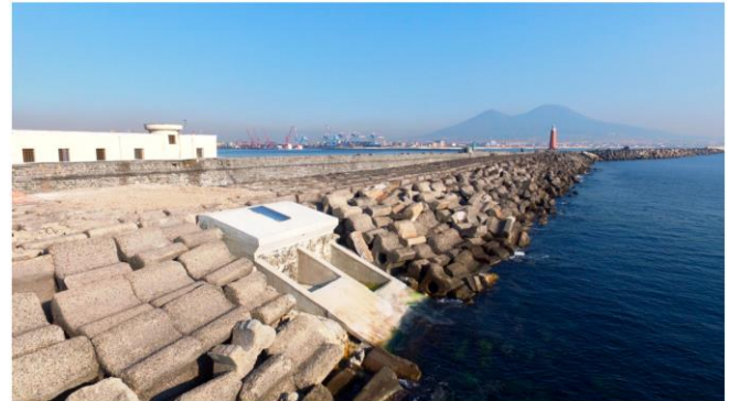
Fig. 1. OBREC prototype installed in the port of Naples (Italy).
