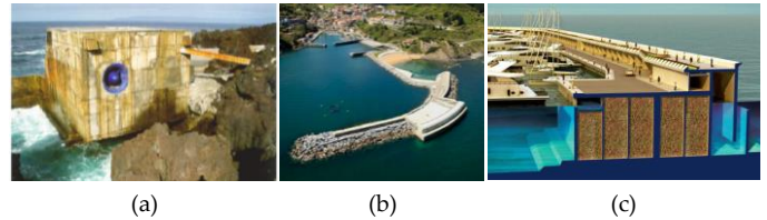
Fig. 1. Examples of OWC: (a) Isolated OWC (Pico, Azores) [9], (b) Mutriku OWC plant [2], (c) REWEC3 3D representation.
