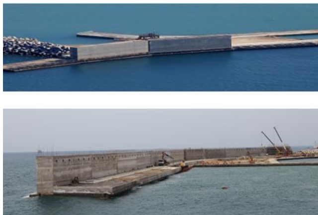
Fig. 2. REWEC3 prototype at Civitavecchia port. First panel (on the top): May 2014. Second panel (on the bottom): September 2016
