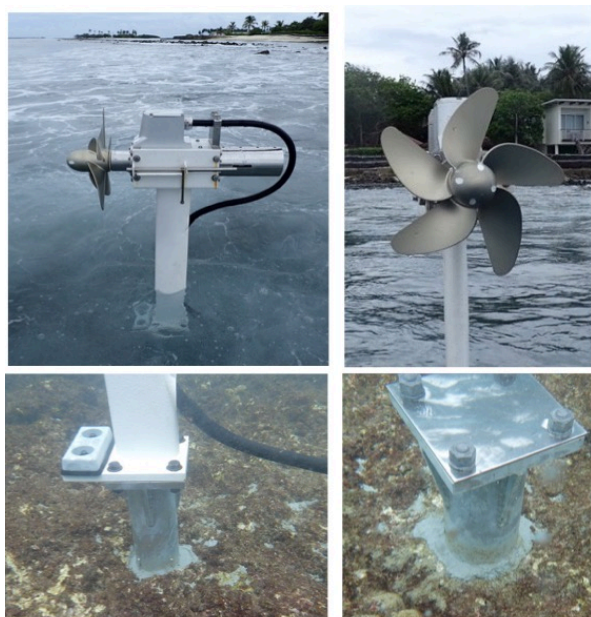
Fig. 5. After drilling the holes, we inserted the sockets, and filled the gap with ceramic-balls, then sealed with epoxy cement on the top. Then we mounted the WEC support, by inserting it into the socket. The square block in the bottom left photo is the zinc anode to reduce rusting.
