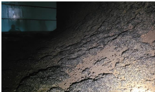
Fig. 7. Attachment of mussels to seawater outflow structure.
