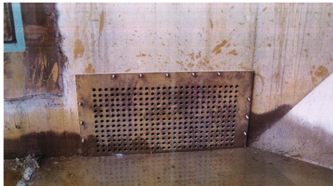
Fig. 2. Drainage screen. There is a drainage screen on the wall below the seawater inlet. During a major inspection, the water in the aqueduct is drained through this drainage screen, but this is difficult due to the adhered mussels.
