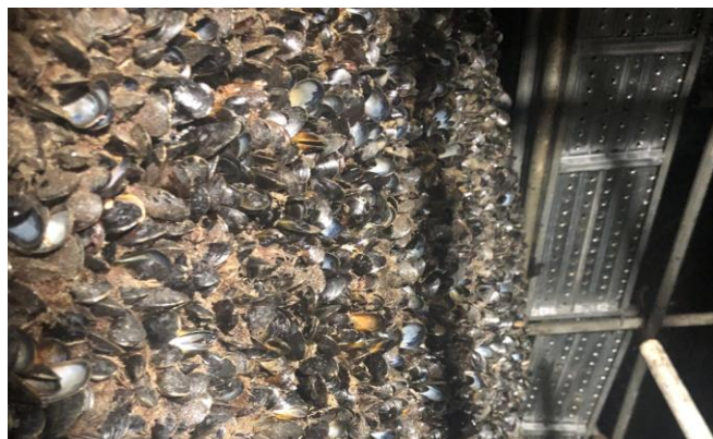
Fig. 3. Attachment of mussels to bulb case.
